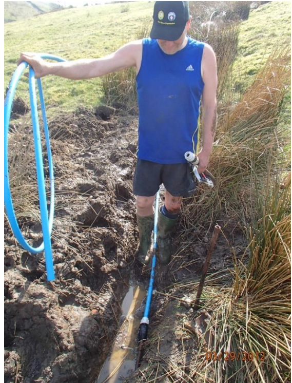
The new pipe Photo Credit: Ray Duffy
