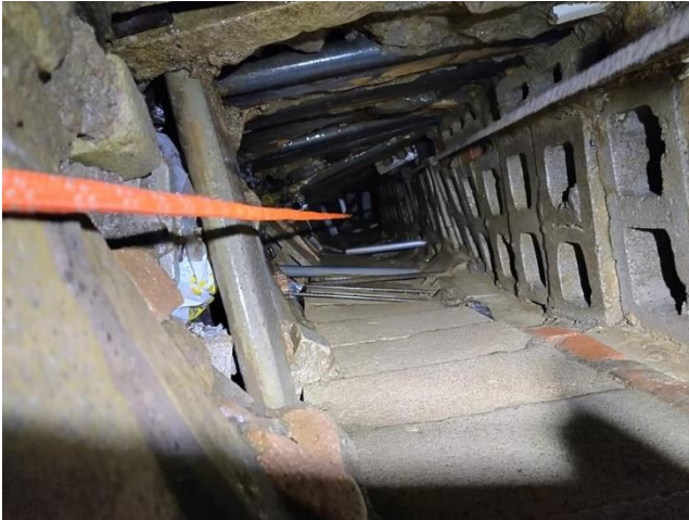
Clever breeze block foot and hand holds in the entrance shaft. Photo: Colin Jones
